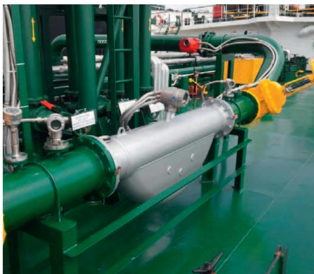
**Bunkering** Bunkering refers to the process of fuelling vessels for their motive power. Currently this is usually fuel oil and marine diesel but in the near future it will be extended to LNG (liquefied natural gas).
